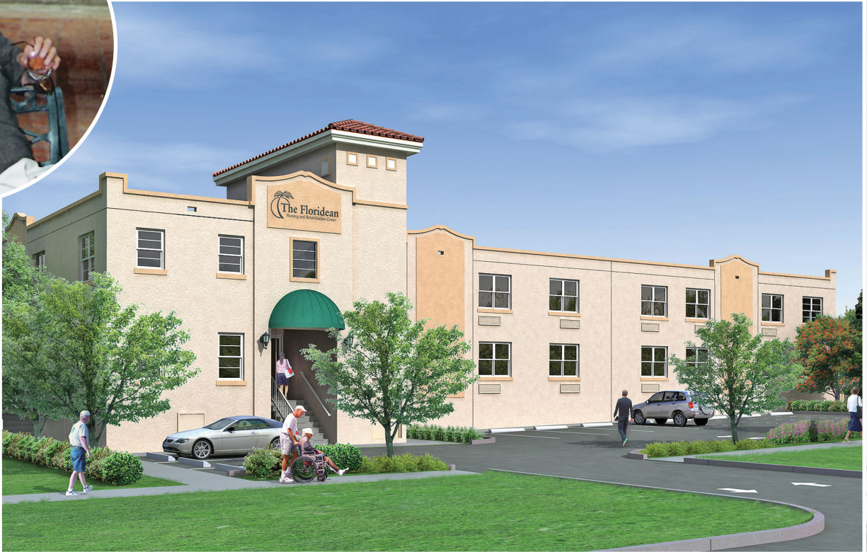
2007 The "Butch Rice" Rehab and Wellness Center at The Floridean. Construction to begin early 2007.
